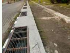
Paved pedestrian path with integrated drainage system
