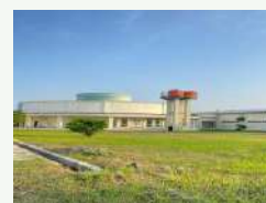
Water tower — gravity-based centralized distribution system
