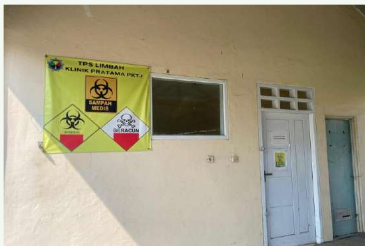
Temporary Hazardous Waste Storage Facility (TPS B3) — PKTJ Tegal
