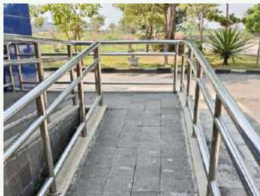
Accessible ramp with handrails — inclusive mobility for persons with disabilities
