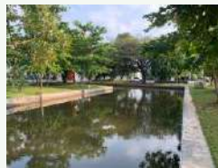
Dormitory wastewater drainage system
