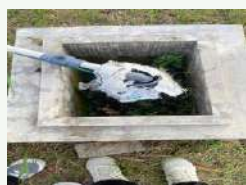
Absorption/infiltration wells — groundwater recharge & runoff reduction
