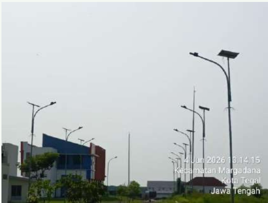
Solar monocrystalline street light (100–150 Wp each, LiFePO4 battery)
