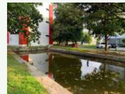
Dining room 3-stage wastewater treatment
