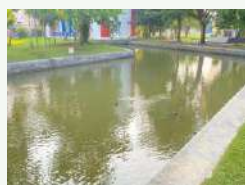
Water retention pond — natural storage & flood prevention
